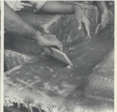
Excess resin and voids are squeegeed out of each lamination.
