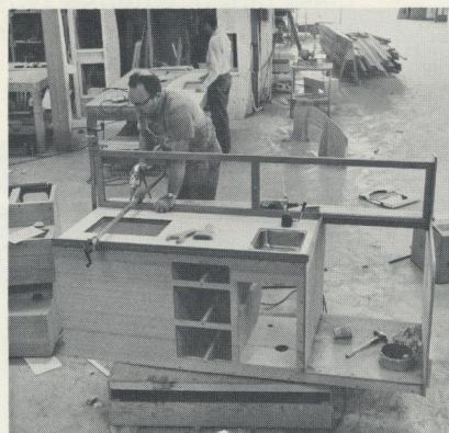
Preassembling the interior permits finer, more efficient cabinet making.
