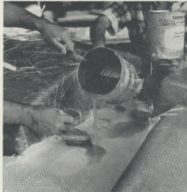
Resin follows fiberglass, poured on and brushed into the weave.
